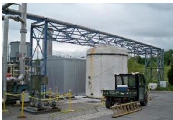
Figure 3.10. The Chromium Water Treatment System
